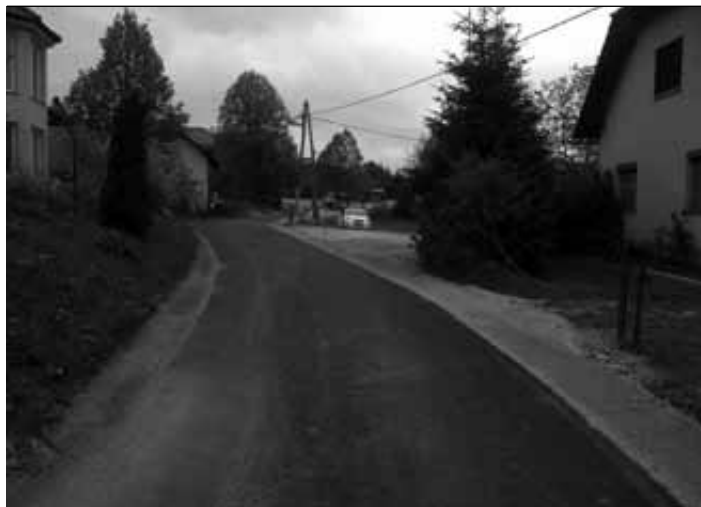
Nov asfalt v Zapotoku
