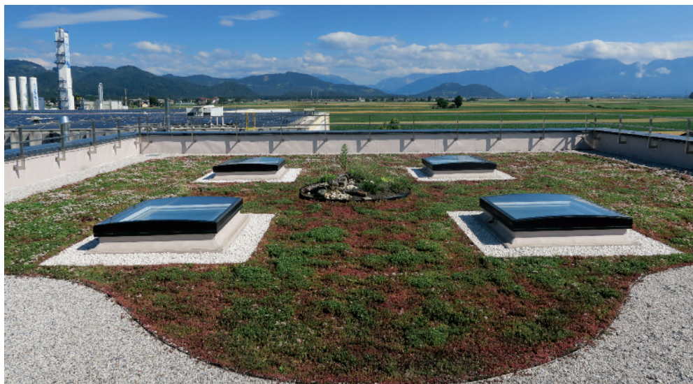
Figure 2: Green roof in Škofja Loka.
