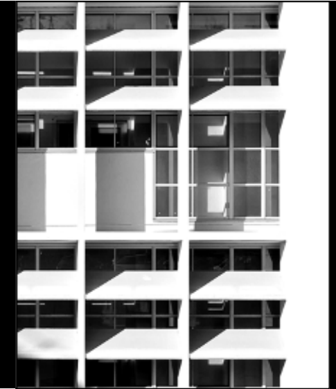
Fig.6: Facade of Officine ICO, one of the additions by Luigi Figini and Gino Pollini (photo Gianluca Giordano).
