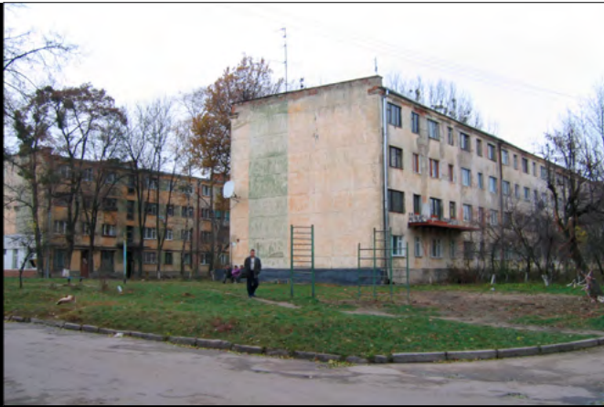
Fig. 1: The first quarter with typical multi-storey buildings on the Pasichna street in Lviv, built in the late 1950s under the design of L. Nivina and S. Dorosh (photo: O. Morklyanyk).
