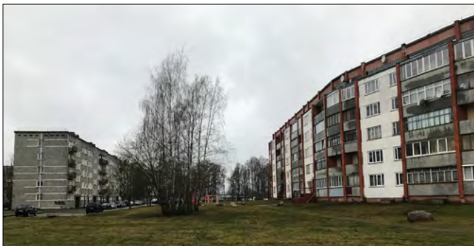
Fig. 10: Brick and reinforced concrete panel buildings in Salaspils (photo by author).
