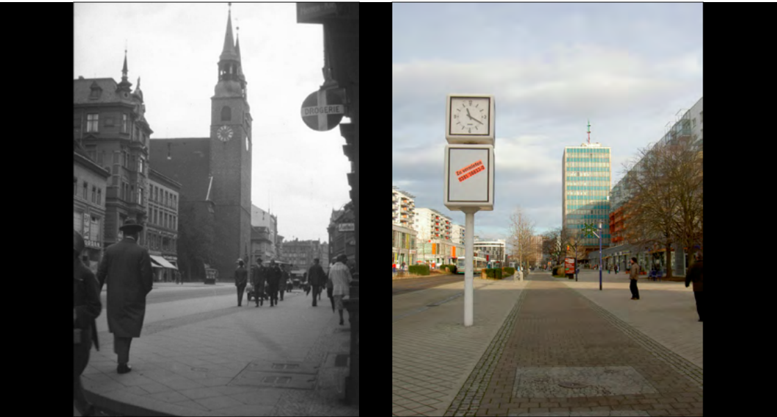
Fig. 7: Magdeburg. St Catherine's Church before demolition in 1964–1966 (photo by Berit Wallenberg / public domain).
