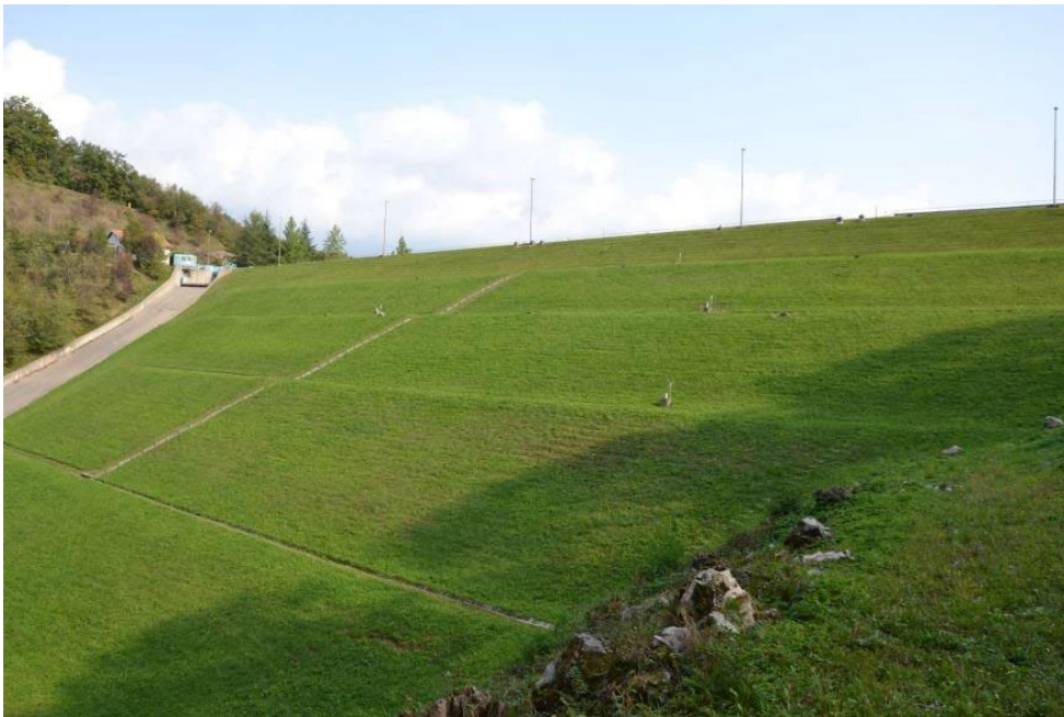
Figure 1. The downstream view of the dam.
