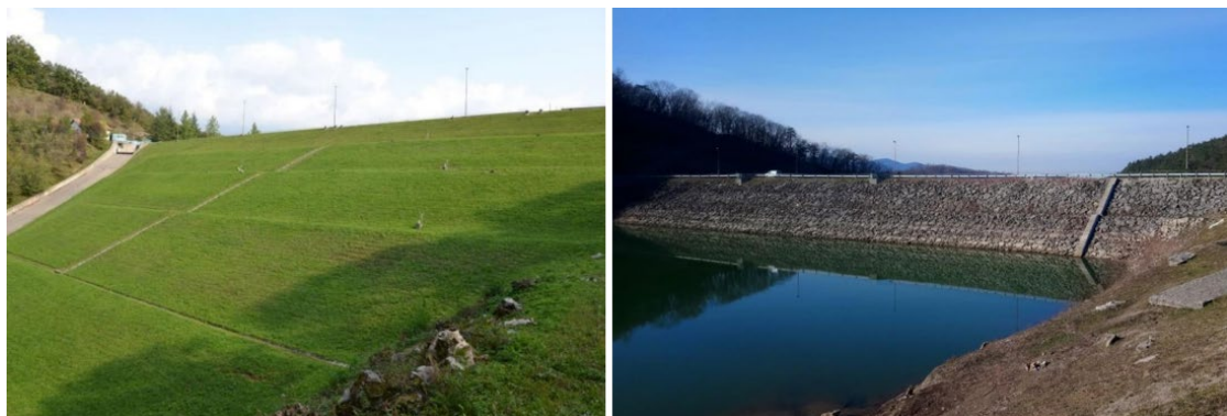
Figure 1. Downstream and upstream face of the embankment dam.
