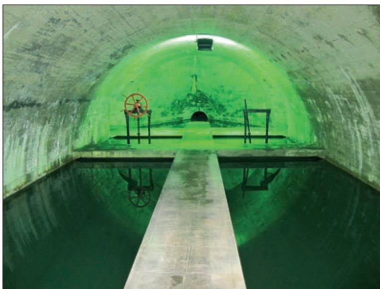
The so-called “Military Water Supply System” was built simultaneously with the public, civil water supply system. It lifted water from the Sv. Ivan spring by means of two piston pumps by as much as 950 m (which due to exceptionally high pressures is rare even nowadays) to the Žbevnica reservoir, and then utilised gravity to supply the then border area all the way from Hrpelje – Kozina to Klana and Mučići.
