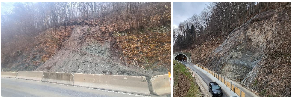
Figure 1: Initial situation of the landslide hazard on the E652 near Tržič before (left) and after (right) the urgent remedial measures (Foto: DRI).
