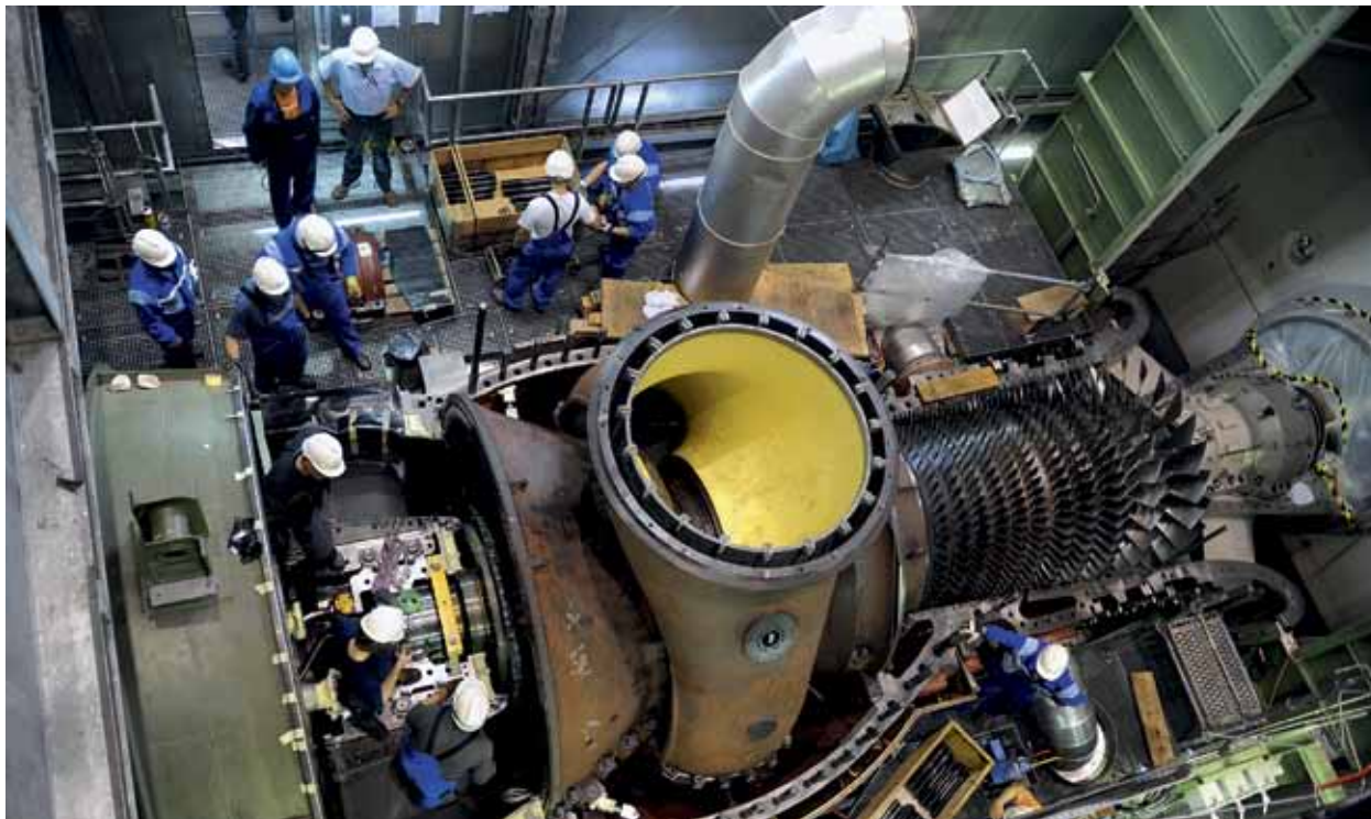
Rotor plinske turbine GT11N2
