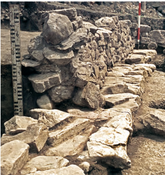
Sl. 25: Hiša 1. Severovzhodni temeljni in drenažni zid; pogled s severozahoda. Fig. 25: House 1. Northeast foundations and drainage wall; view from the northwest.
