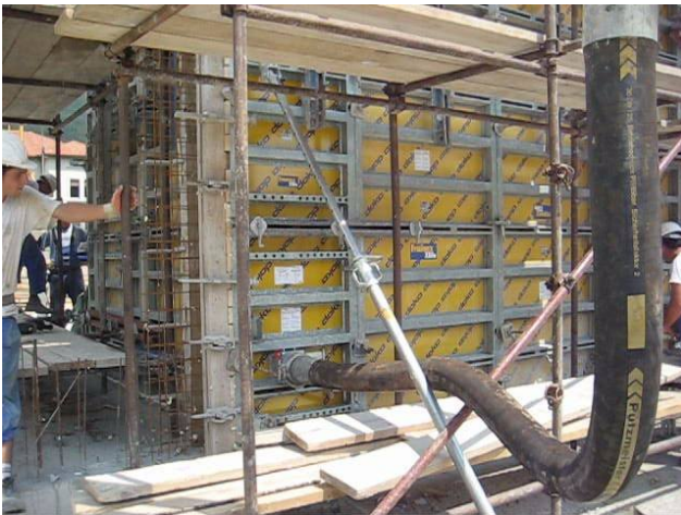
Figure 13: Casting of slender walls by pumping of SCC bottom up.
