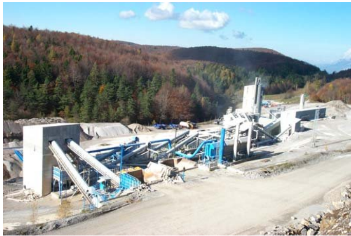
Figure 4: Separation plant with several silos for limestone filler.
