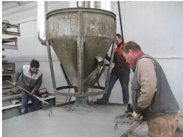
Figure 7: Casting of element in the Laže precast plant.
