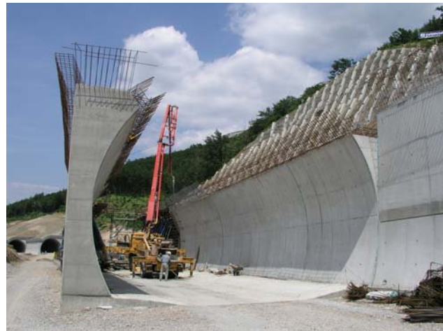
Fig. 14: Heavily reinforced cut-and-cover tunnel on the motorway Razdrto-Vipava.
