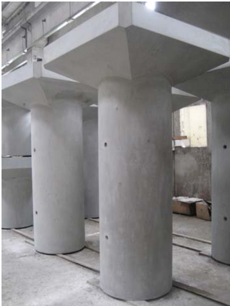
Figure 10: Hollow caps for steel piles.
