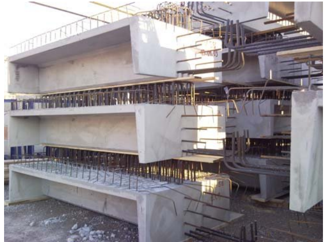
Figure 9: Elements for the construction of piers.
