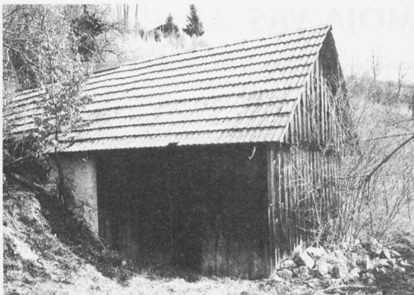
Preprosta zidanica z leseno lopo pred zidanim delom
