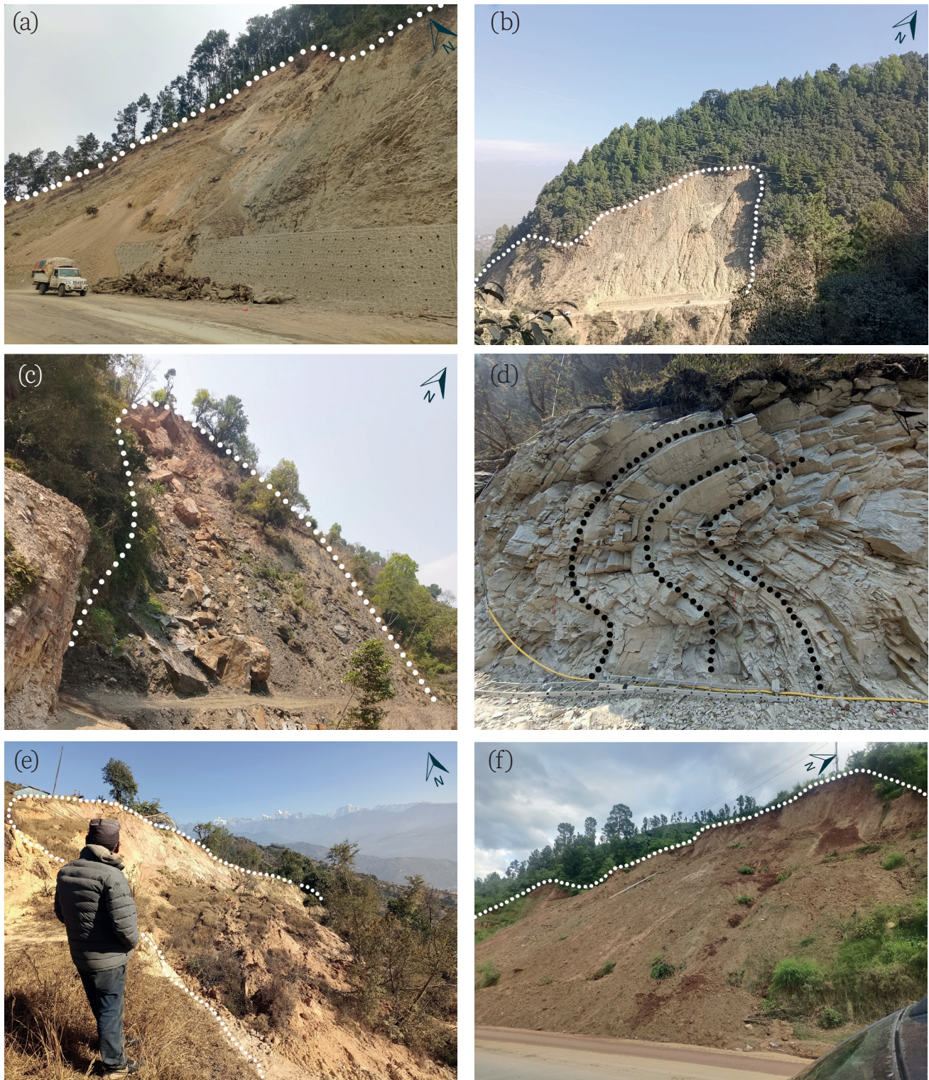
Fig. 2. Cut slope characteristics in the Lesser Himalayan Zone of western and central Nepal: (a) weak rock exposure and steep cut slope failed during heavy rainfall along the Prithvi Highway, Tanahun, (b) completely weathered high slope along the Kanti Lokpath, Lalitpur, (c) rock blocks over loose materials failed along the Pushpalal Highway, Kaski, (d) folded rock showing numerous discontinuities prone to failure at Dolakha, (e) a translational slide along the Kathmandu-Melamchi Highway, Sindhupalchowk, and (f) a failed residual soil slope due to slope modification for highway expansion along the Prithvi Highway, Dhading.
