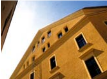
Slika 1: Masiven značaj fasad mlina je ohranjen. The massive character of the mill elevations has been preserved.
