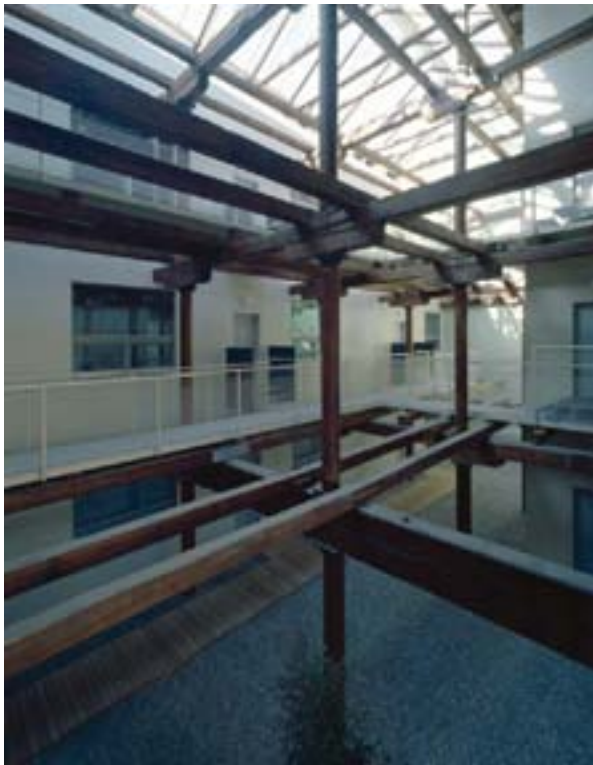
Slika 3: S projektom se v dvorišču, prekritem s stekleno streho, lesena nosilna struktura razkrije v obliki prostorske mreže. The project exposes the wooden construction as a spatial grid in the court covered by a roof light.
