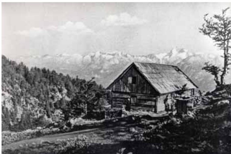
Figure 5: The Orožen hut on the Lisec mountain pasture under the summit of Črna prst was the first mountain hut built by SPD. It was built in 1894, one year after SPD was established. The hut was built of thick plates and covered with shingles. Its length was 11.5 meters, while the width and height measured 6.5 meters. There was an entrance porch under the roof and they assumed it would be sufficient for accommodating twenty people. The opening was very festive and magnificent, and the event was quite important for that time. The guests were welcomed by an inscription saying “The first mountain hut opens, the entire valley of Bohinj rejoices!” in Bohinjska Bistrica. Photo archive: Peter Mikša.
