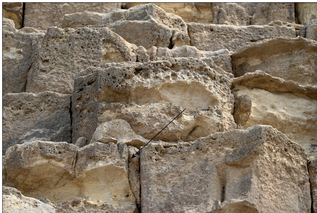
Figure 35: Binding material between stone blocks and a recess in the middle of a stone block. Width of view is 4 m.
