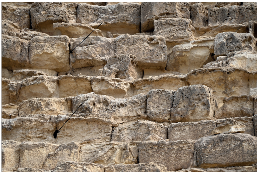
Figure 32: Hollows and channels at the contact points of stone blocks. Width of view is 9 m.
