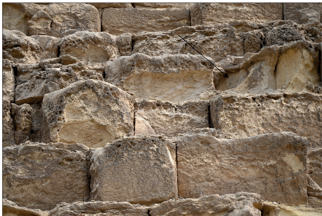
Figure 33: Hollow next to a vertical fracture. Width of view is 6 m.
