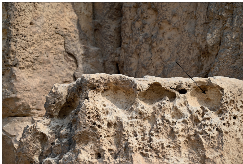
Figure 37: Flaking of cups circumferences. Width of view is 1.5 m.
