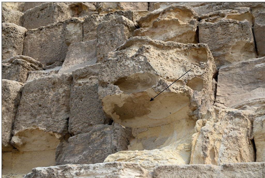
Figure 38: Flaking of cups circumferences. Width of view is 5 m.
