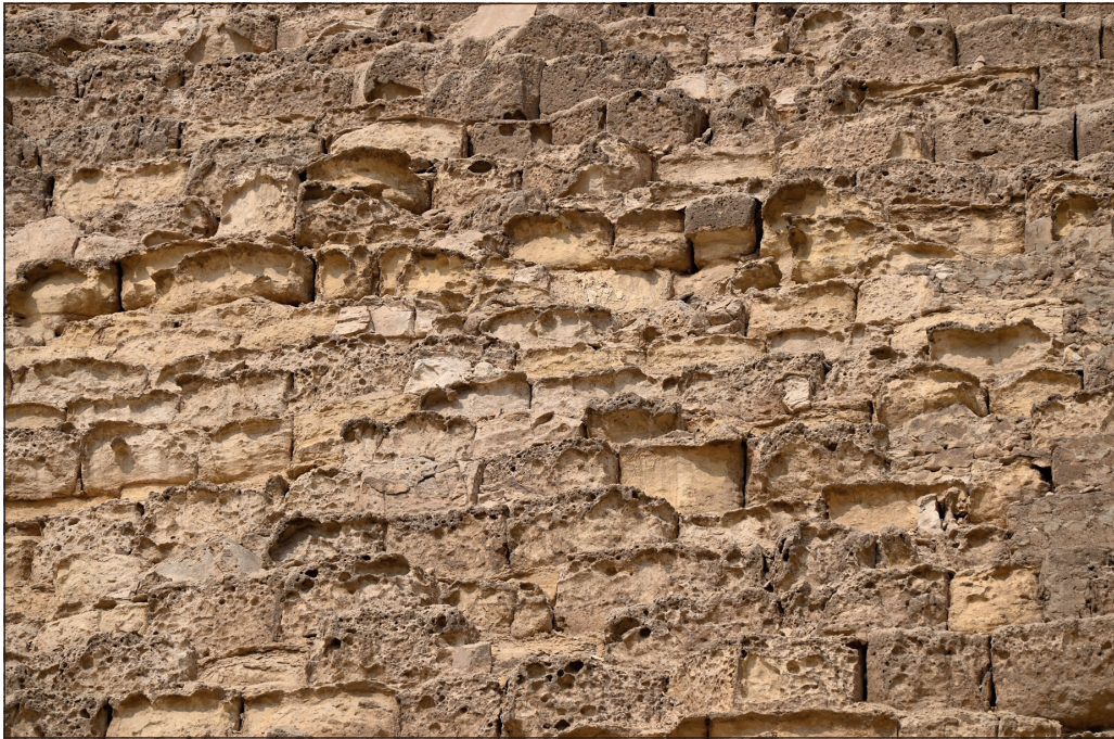
Figure 30: Wind-formed depressions. Width of view is 15 m.
