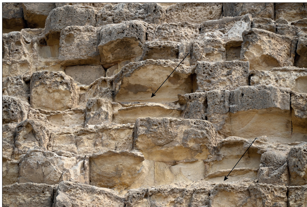
Figure 29: Depressions – traces of wind erosion. Width of view is 8 m.
