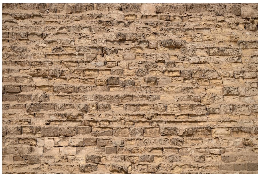
Figure 5: Disintegration of stone blocks on the western side of the pyramid.
