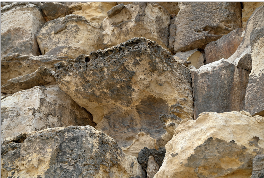
Figure 23: Overhanging rock block with crust cap and below wind cups with flaking surface. Width of view is 4 m.
