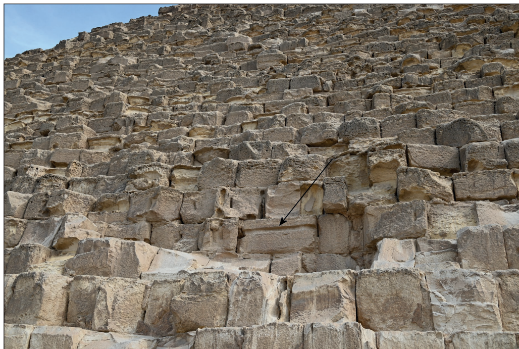
Figure 36: Artificial recess in the wall of a stone block.
