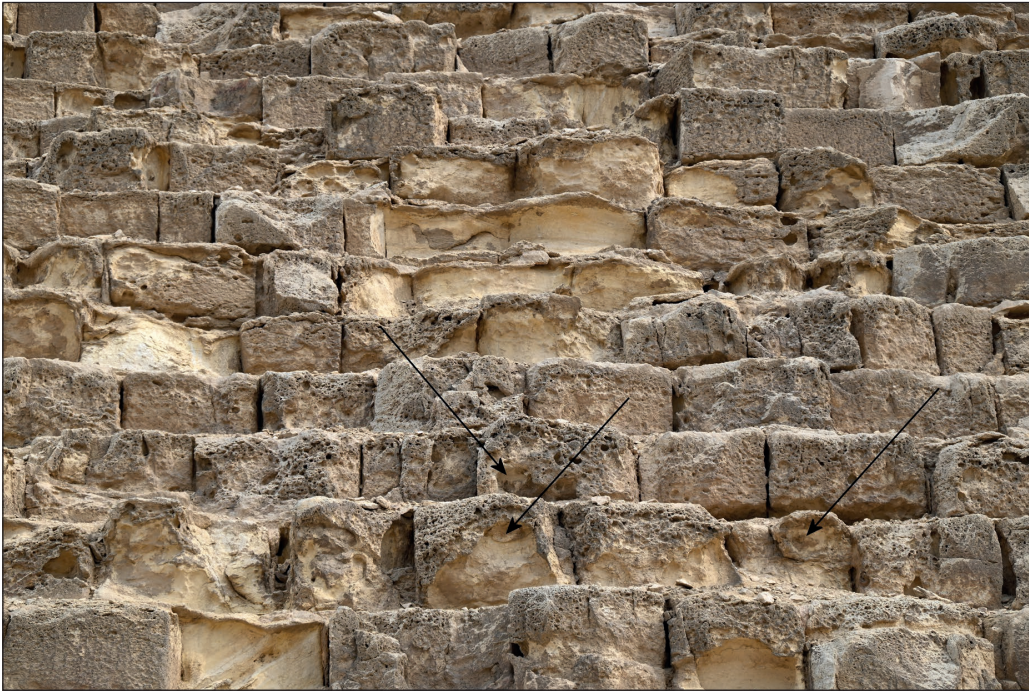
Figure 18: Eroded stone blocks. Width of view is 12 m.
