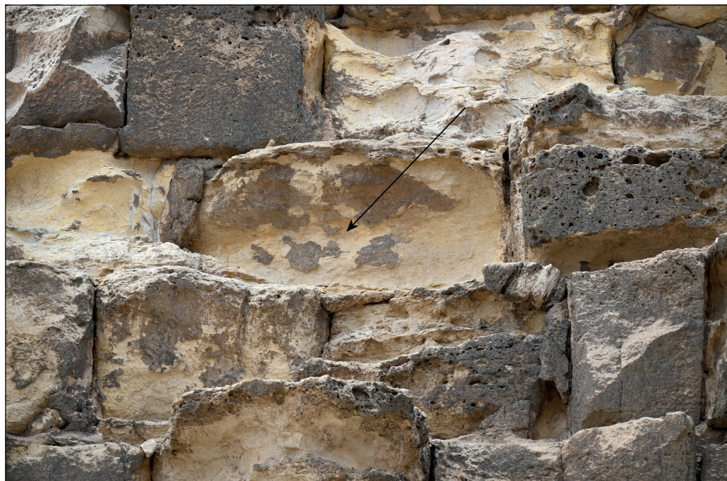
Figure 28: Crust flaking. Width of view is 4 m.
