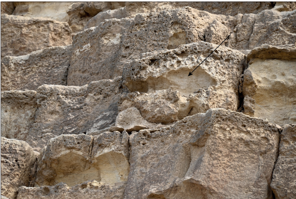
Figure 31: Shallow cups on the ceiling of larger wind-formed recesses. Width of view is 5 m.
