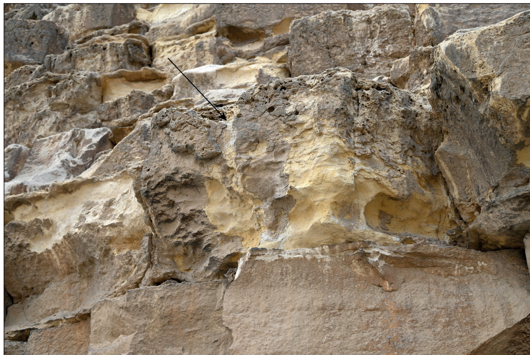
Figure 26: Traces of water runoff from the top of a stone block and wind cups in its lower part. Width of view is 4 m.
