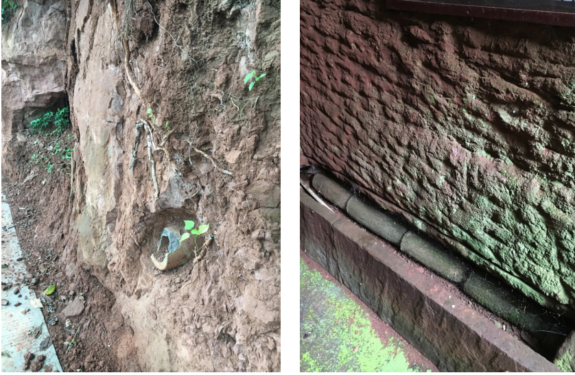
Figures 5a, 5b: Cliff tomb drainage pipes, Pengshan, Sichuan (Photos by Author).
