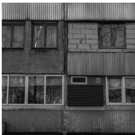
Figure 5: Inadequately renovated facade of Jugomont's residential building JU-61.
