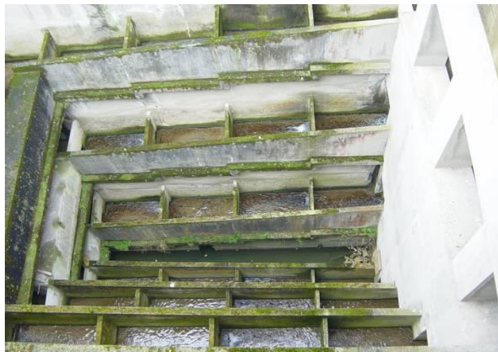
Slika 18: HE MB otok – pogled na ribji prehod od zgoraj. Figure 18: HPP MB otok – fishway view from the top.
