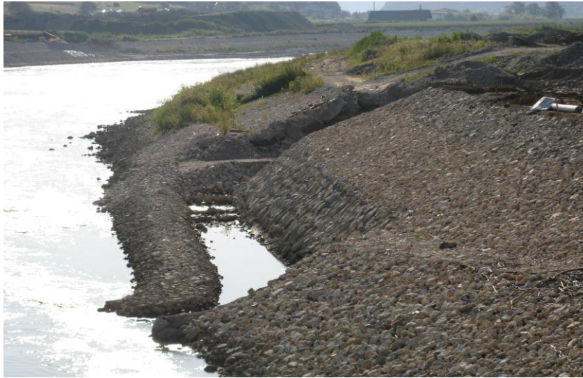
Slika 4: HE Blanca – vhod v obhodni kanal. Figure 12: HPP Blanca – entrance to bypass fishway.
