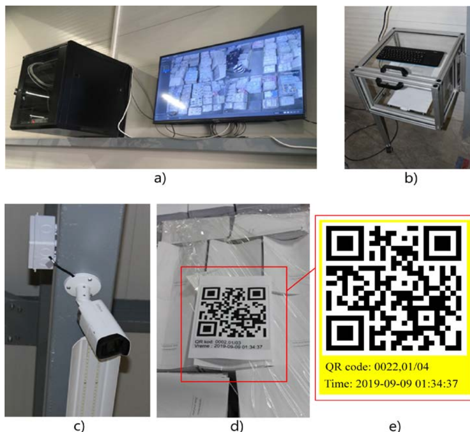
Fig. 5 Preview of the implemented solution: a) Large screen and server (including PC, switch and NVR device) placed in the protective box; b) Printer placed in the protective box; c) Dahua 8MP IP camera mounted on the roof construction; d) QR code placed on the top of the pallet; e) QR code format
