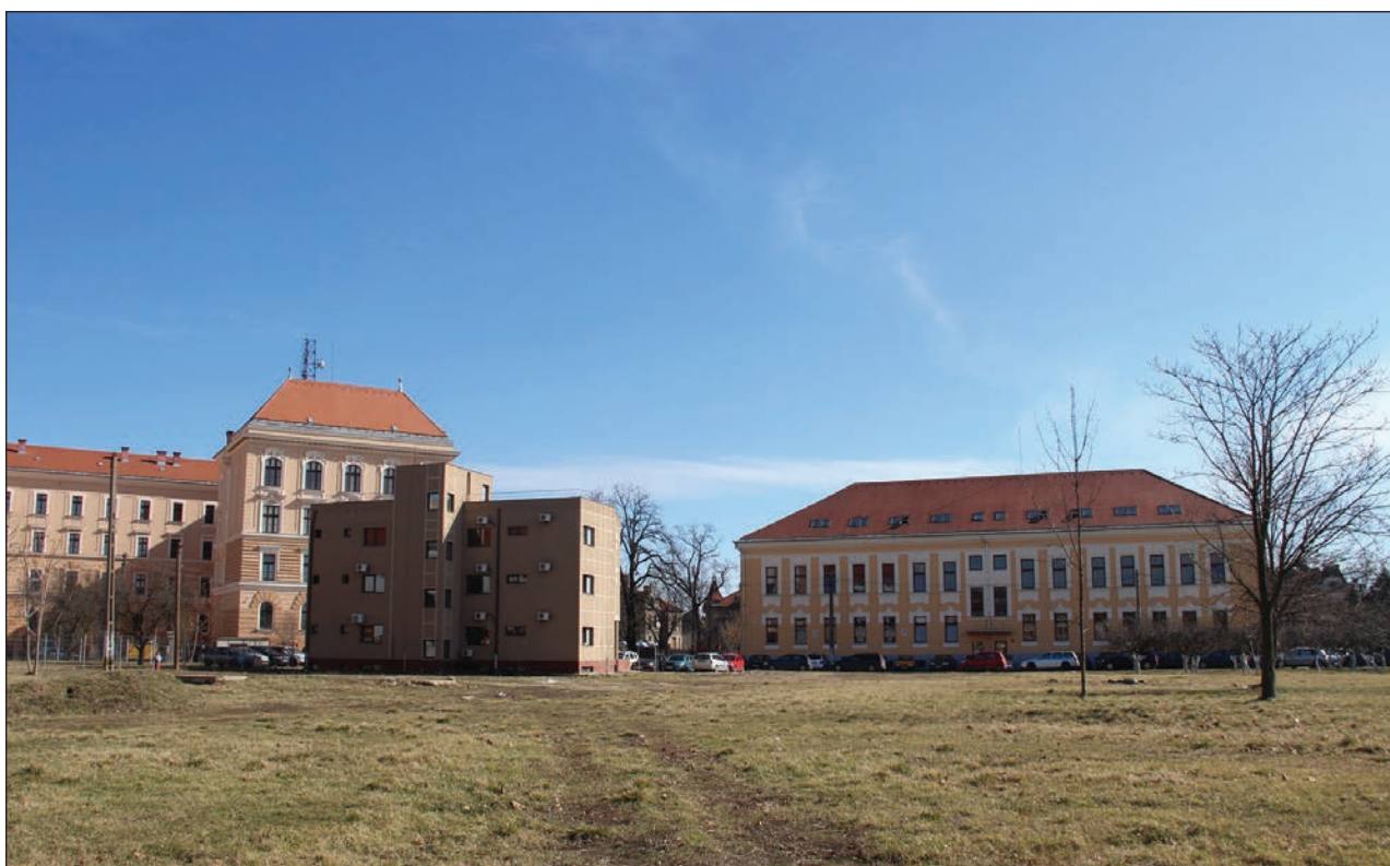
Figure 19: Renovation and transformation of the former military facilities (Source: the authors).
