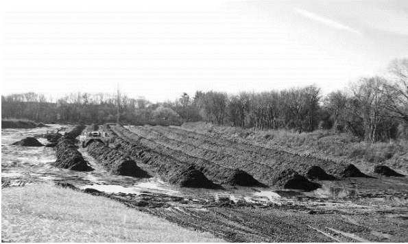
Figure 2: Windrow composting. (Greenville County Soil and Water Conservation District, 2019)
