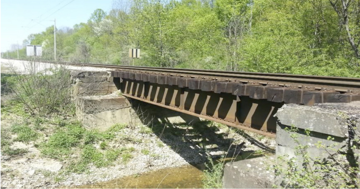
Figure 1: Old steel bridge.
