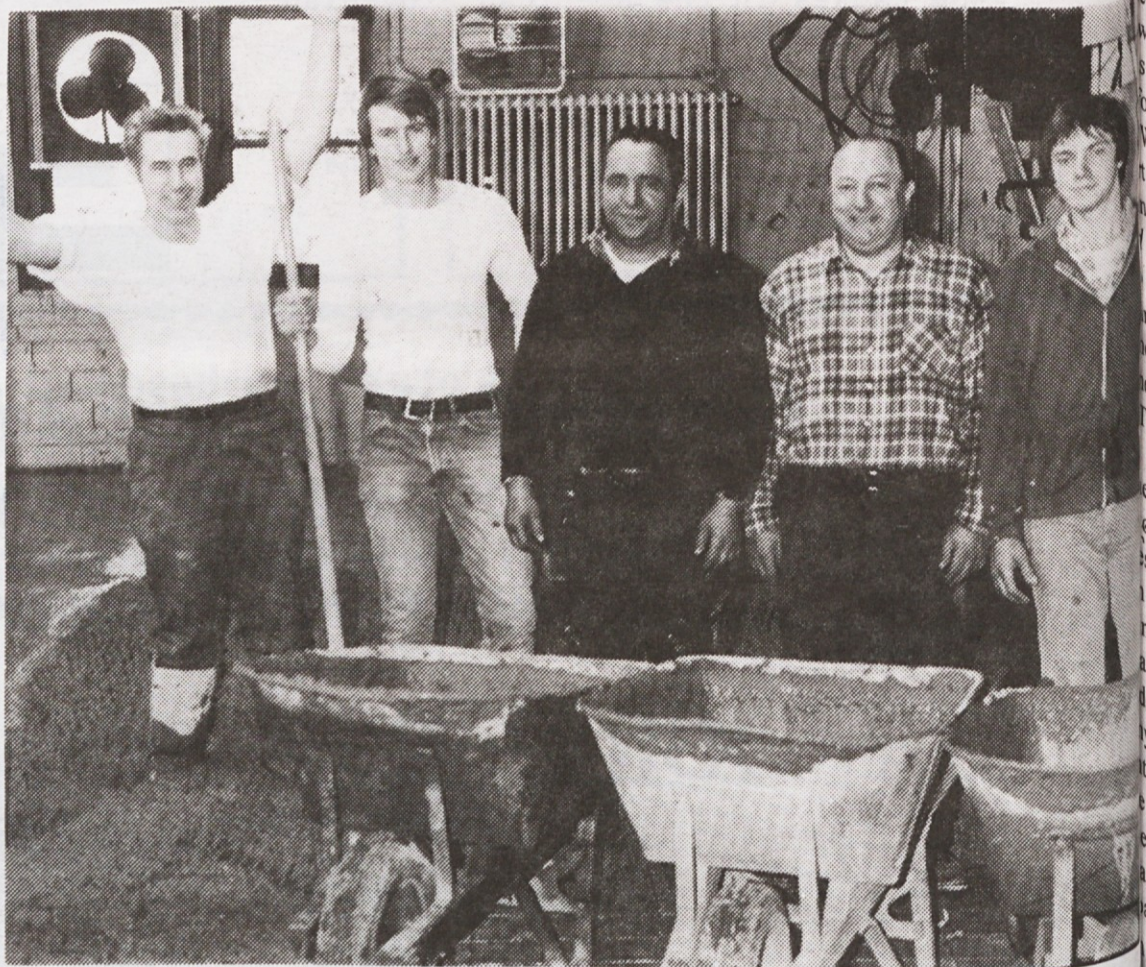
The floor of the American Home Publishing Co. had to be removed and 8 inches of concrete poured to hold the new off-set printing press purchased in 1983. Donating their time, talent, and cement were, left to right, Joze Omahen, Joseph J. Omahen, Alojzij Fortuna, Nance Omahen, and John Grm, Jr.
