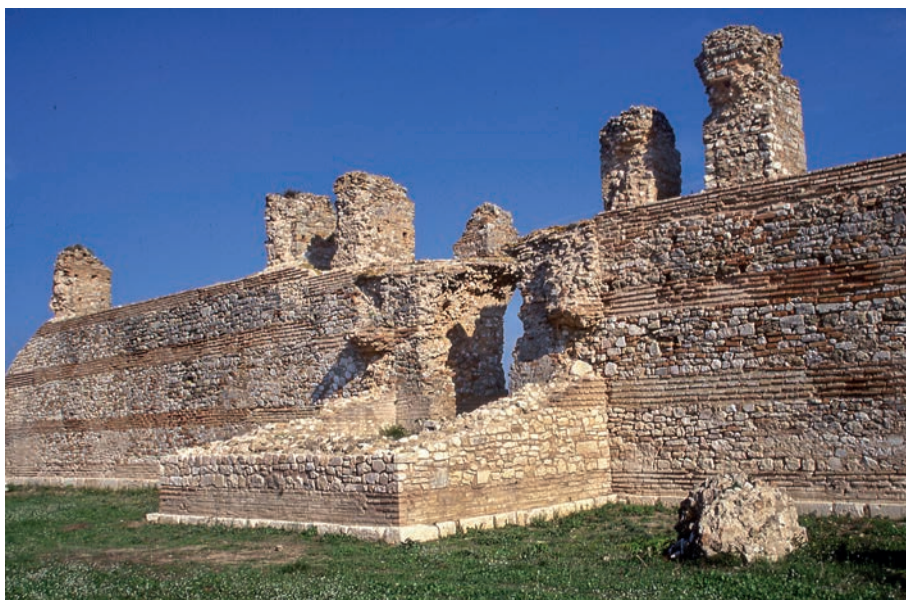
Fig. 2.146: Nicopolis. Well-preserved city wall from the south (2002).
