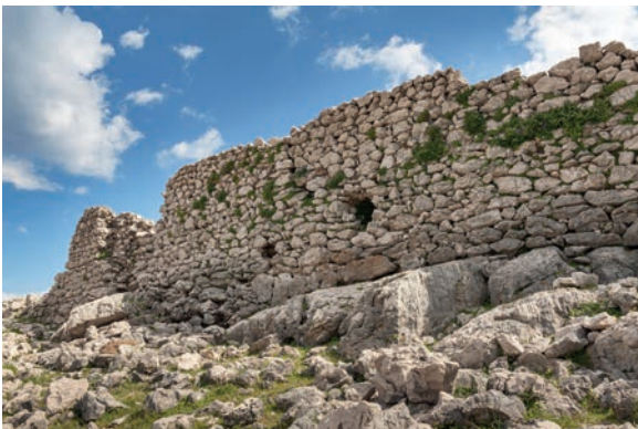
Fig. 3.149: Korintija near Baška. Walls from the north-western part of the fortification (2021).
