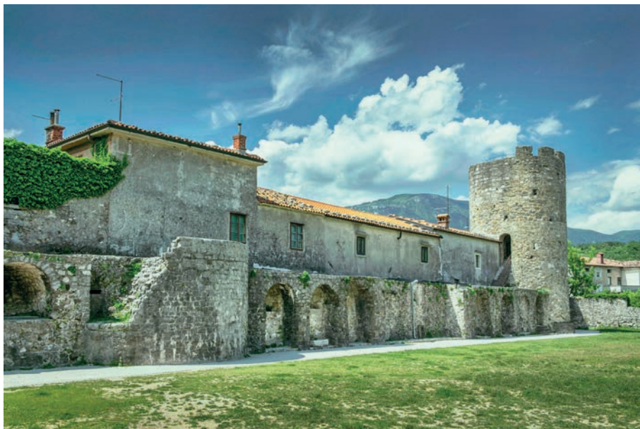
Fig. 3.99: Ajdovščina ( Castra ). Eastern walls with a tower (2015).
