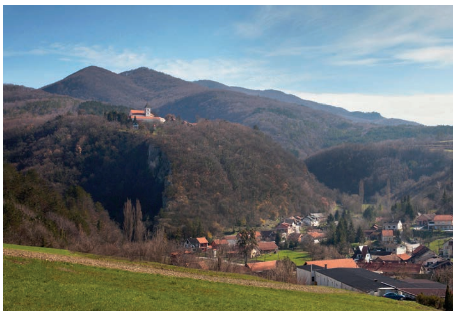
Fig. 3.135: Marija Gorska near Lobar. Fortified settlement from the south-west (2017).
