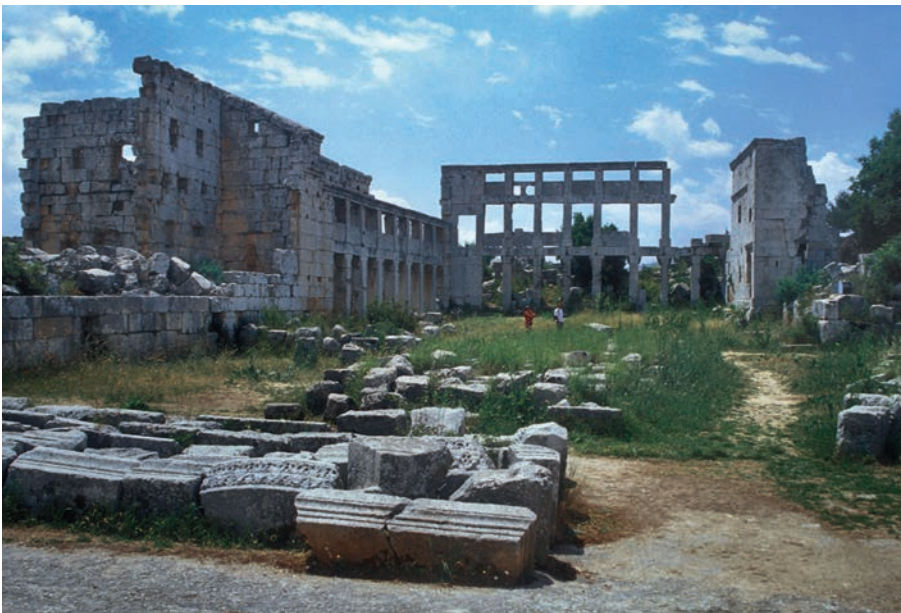
Fig. 5.68: Qalaat Samaan. Monastery in a pilgrimage centre, preserved to a substantial height (2004).
