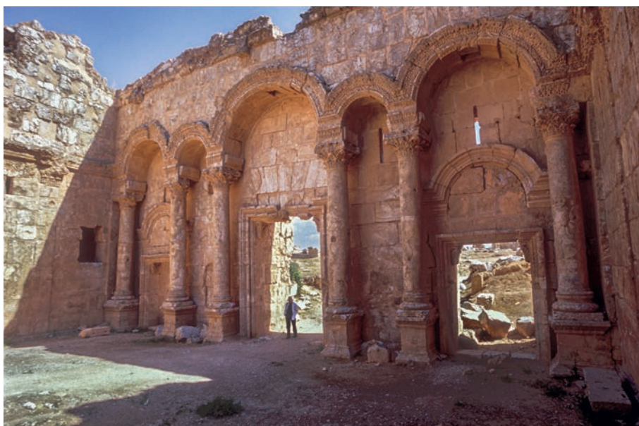
Fig. 5.41: Sergiopolis (Resafa). Ornate facade of the north entrance to the city (2004).
