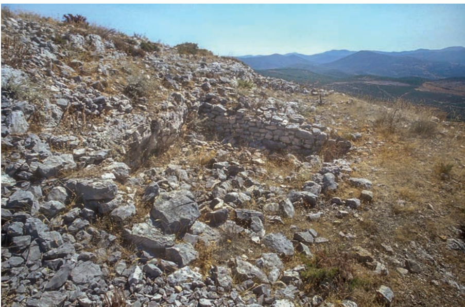
Fig. 2.64: Municipium Ridentarum. Remains of a Late Antique building cut into the bedrock (2006).
