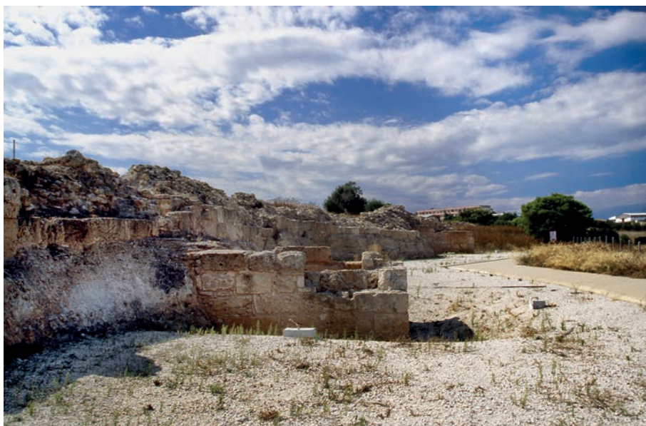
Fig. 3.298: Isthmia. Well-preserved barrier wall of Hexamilion near the fortress (2007).
