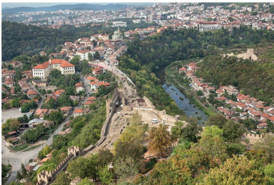
Fig. 2.203: Carevec. View from the top of the city towards the entrance in the west (2012).
