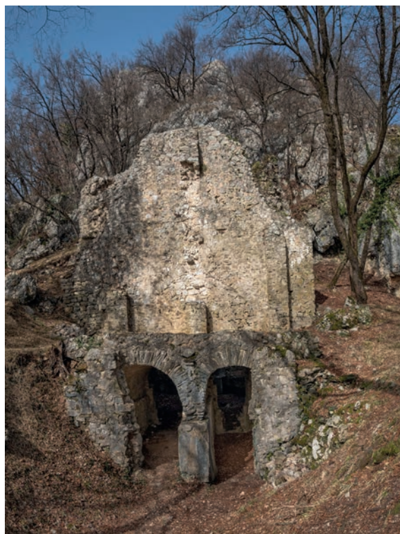
Fig. 3.94: Sv. Pavel above Vrtovin. Tower above the spring on the southern foothills of the hilltop site preserved to a great height (2021).
