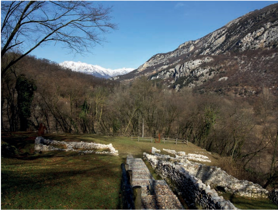
Fig. 3.60: Sant'Andrea di Loppio. Remains of the buildings in the north-western part of the fortification (2016).
