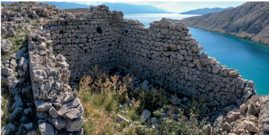
Fig. 3.148: Korintija near Baška. Cistern preserved to a great height in the south-eastern part of the fortification (2021).
