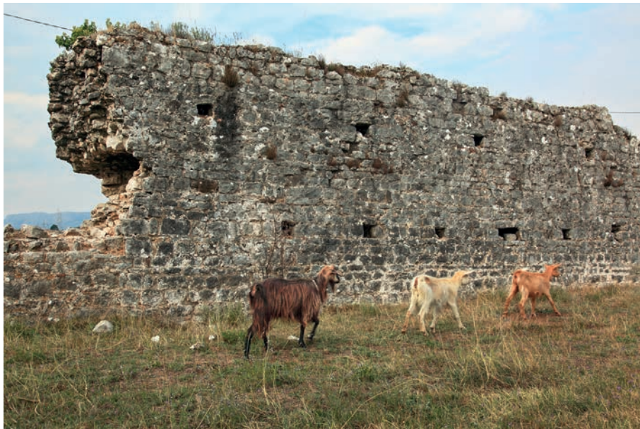
Fig. 2.80: Doclea. City walls preserved to a substantial height (2009).
