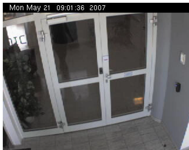
Figure 1. A case access point: the door opens when two sensors on the right side confirm the identity of the acceding person. The upper sensor is an identity card reader and the lower a fingerprint reader.
