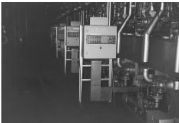
Slika 1: Plinski gorilniki ter krmilna elektronika Figure 1: Gas heaters and regulation electronics
