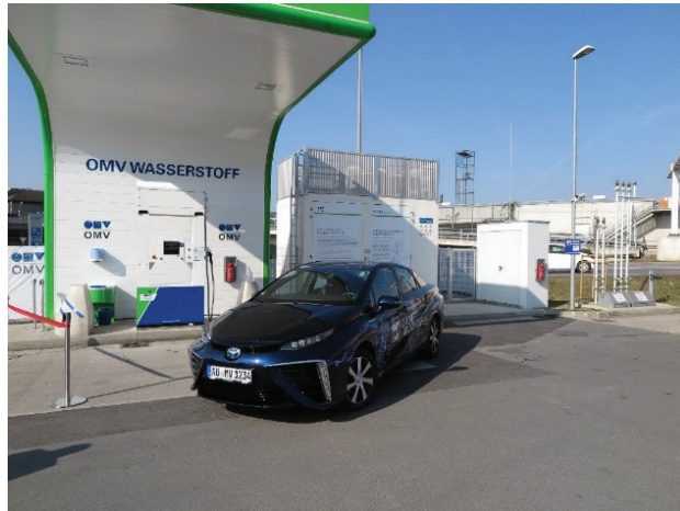
Figure 7: Hydrogen fuel station with Toyota Mirai car
