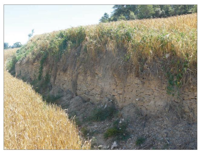
Figure 5: Stone wall not reaching up to the surface of the upper field. Notice soil sediments accumulated at the base.
