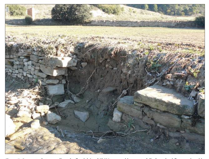
Figure 7: Segment of stone wall on the floodplain of El Sió removed by a waterfall of overland flow produced by the storm of 2nd November 2015 (c. 75 mm in 3 h). Notice the volume excavated by the waterfall at the base of the missing segment of the wall.
