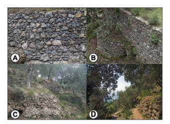
Figure 8: Dry-stone walls in conglomerate:
