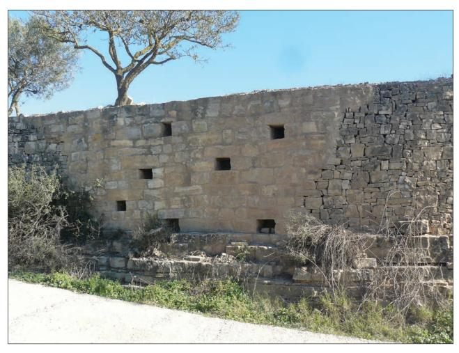
Figure 3: Stone wall built on a limestone outcrop with repaired segment on the left (notice drainage holes) and old segment on the right.
