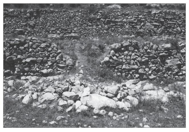
Figure 10: A collapsed wall landslide.
