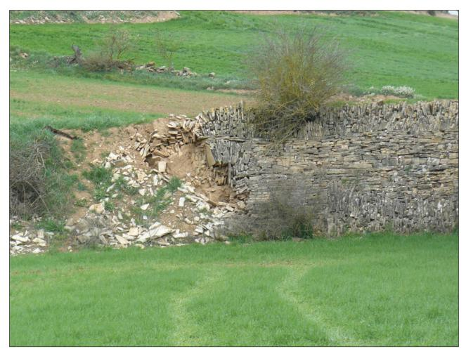
Figure 2: Dry-stone wall with derelict segment (on the left) and standing segment (on the right) with three to four different patterns in the structure.
