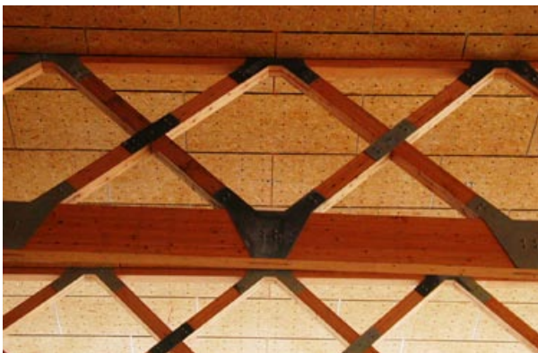
■ Slika 6. Detajl montiranega nosilca Figure 6. Detail of girder as placed
