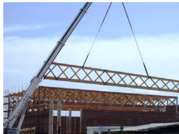
■ Slika 9. Montaža nosilcev z avtodvigalom Figure 9. Erecting of trusses by auto-crane
