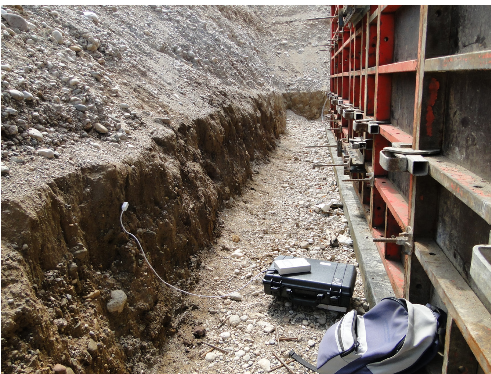
Fig. 4. Field measurement of the thermal parameters with the KD2 Pro meter.
