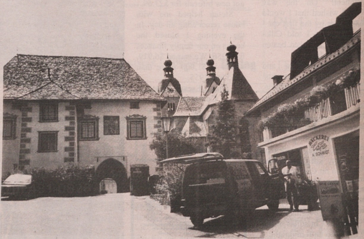
Backside of Cathedral of Gospa Sveta. One of the first Christian churches built in Carinthia, historically considered the first Catholic Church for the Slovenian people. Located approximately 20 miles northeast of the capital city of Celovec, province of Carinthia, now Austria.
