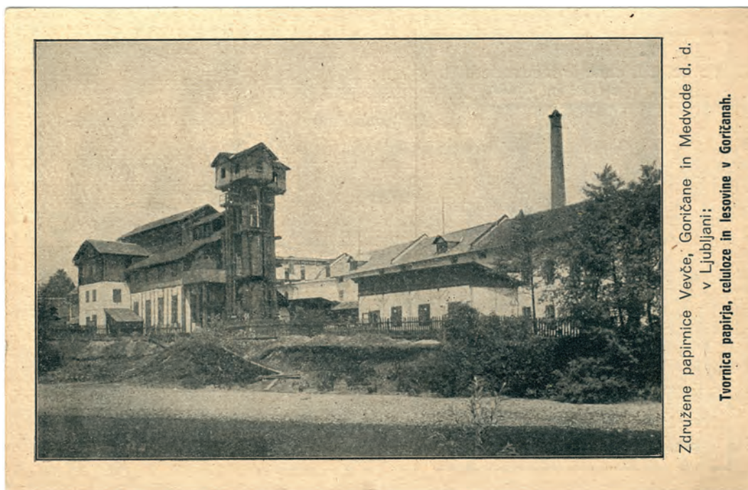
A photo of pulp production as seen on the «island» between the Sora river and the turbine duct.
