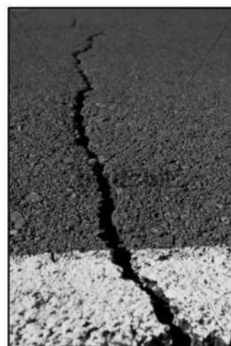
Figure 3: Cracking
