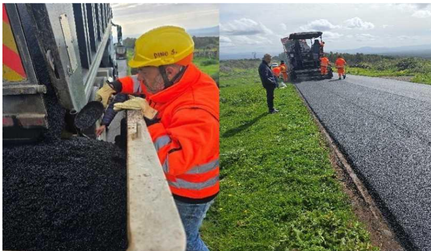
Figure 5. The material during discharging and laying
