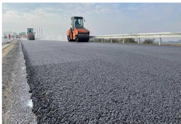
Figure 1. Compaction of the laid asphalt at circa 0°C ambient temperature.
