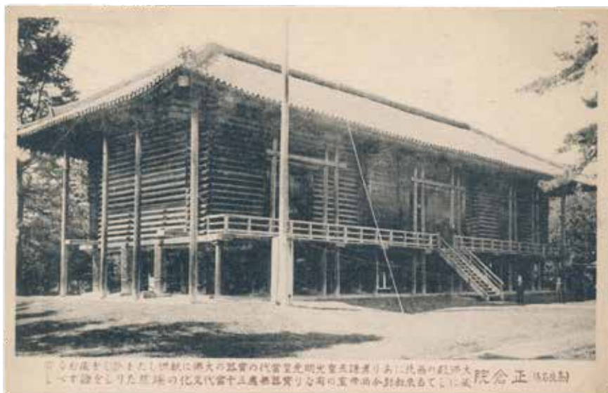
Photo 27: Shōsōin in Nara.
