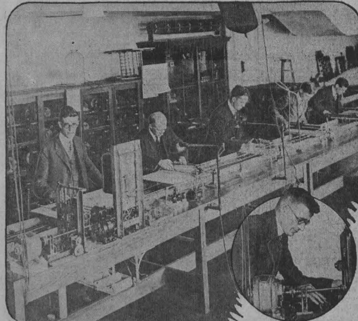
The "product integrator," an electrical machine which thinks for itself, solving mathematical problems too complex for the human mind to master, was the recently announced invention of Dr. Vannevar Bush of the Massachusetts Institute of Technology. Problems in advanced electric theory are worked out faultlessly by the machine. The observers are shown above, watching the operation of moving tables on which are plotted the conditions and equations of a problem. — The insert shows Dr. Bush adjusting the integrator.
