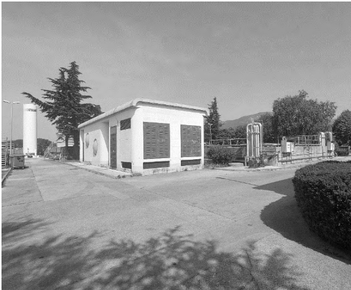
Fig. 6 Cryogenic liquid oxygen storage tank (on the left) and MIXFLO® systems.
