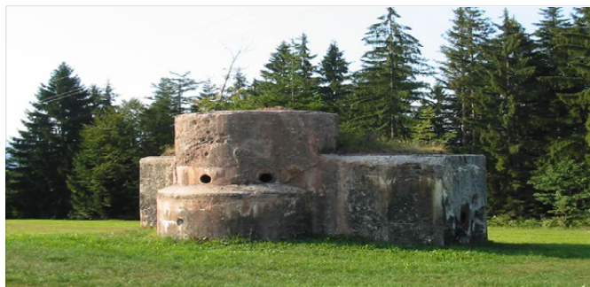
Figure 12: A typical machine gun bunker on Javorč, a symbol of Rupnik defence line (Source: Municipality of Gorenja vas-Poljane).
