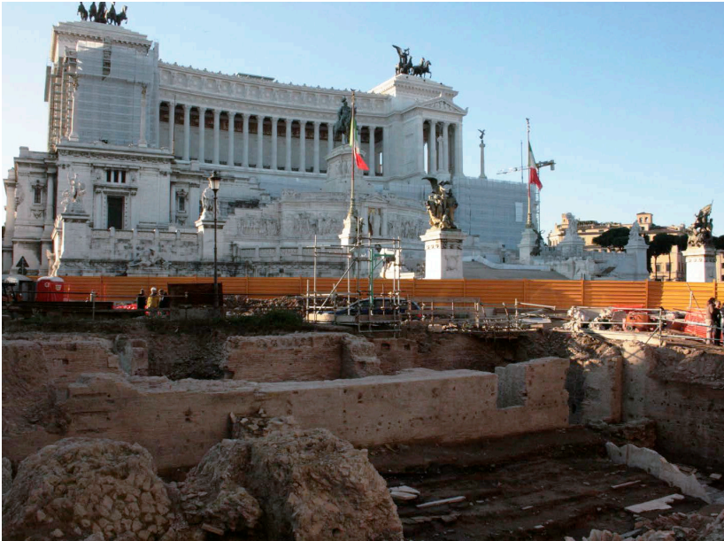
Fig. 2. The so-called auditorium of Hadrian, a horseshoe-shaped structure dating from Hadrian's era, unearthed during preventive archaeology excavations carried out before work began on the construction of the Rome metro line C. Seven years after the end of the excavations, the structure (a public building of great importance) lies untouched with little information provided to the public, in piazza Santa Maria di Loreto, in the centre of the city, just a few steps from the Trajan Column (©Soprintendenza Speciale per il Colosseo e l'area archeologica di Roma).
