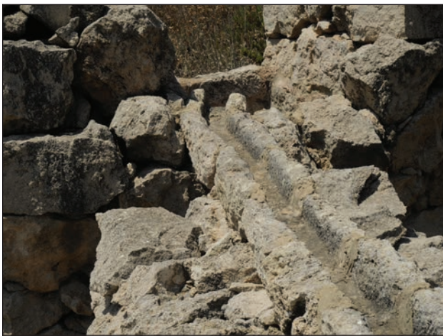
Image 32: The dikes are open for cleaning and for monitoring.
