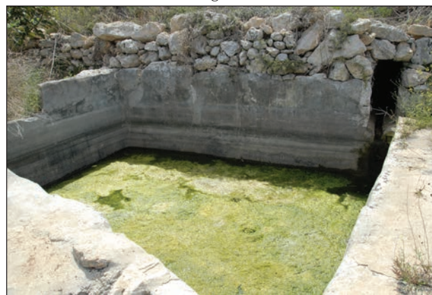
Image 28: A basic object for watering small gardens and fields is a basin. a/ It seems there is a natural water source: there is not. The hole is visible, big enough for a man and for maintenance. An open basin has strong evaporation – this means loss of precious water (1995). The basin is today covered, the inspection hole is surrounded by concrete bricks (2013).
