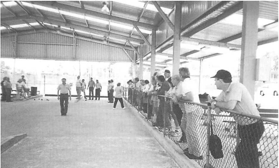
New lanes were built as soon as the club moved to its new premises in Wetherill Park. A shelter was built over the lanes in 1995.
