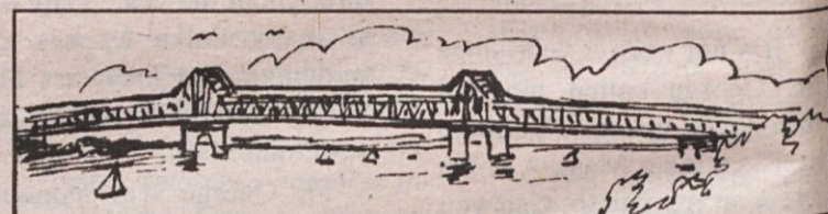
The longest cantilever bridge in the United States is the John Barry Bridge, in Chester, Pennsylvania. It spans the Delaware River and measures 1,644 feet.
