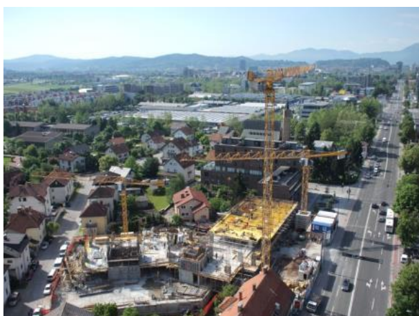
(c) Posnetek gradbišča; perspektiva 1b (c) Aerial photo; perspective 1b
