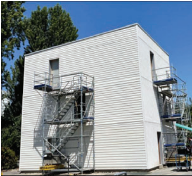
Figure 1: In-situ flanking transmissions measurements facility for high-rise wooden buildings
