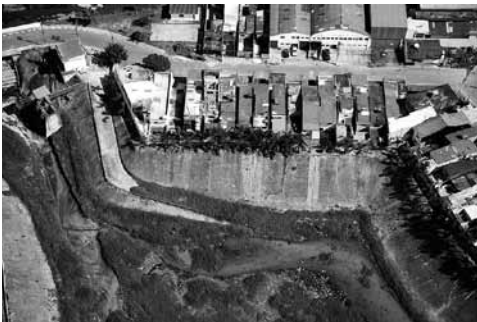
Rezervoar, postavljen tik ob hišah. Reservoir placed right next to people's houses.
