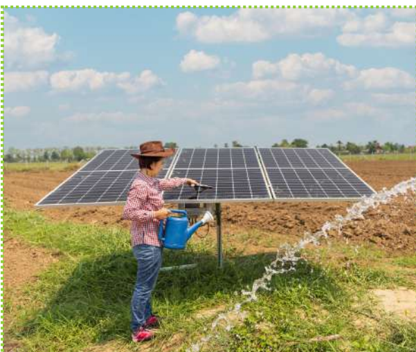
solar panel system
