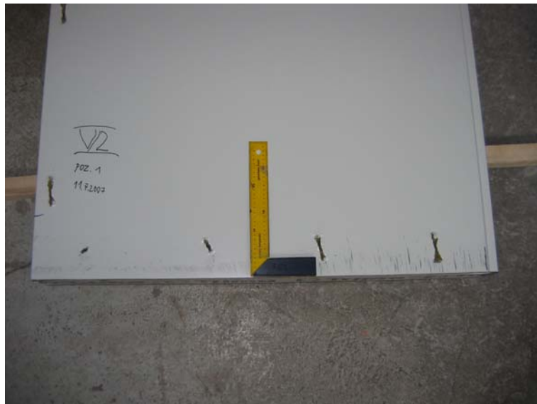
Slika B.35: Pretrg notranje pločevine zunanjega panela Figure B.35: The tear of the inner steel sheeting of the outer sandwich panel
