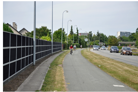
Figure 1. Miljøskærm noise barrier installed in Copenhagen suburb Vallensbaek in 2016.
