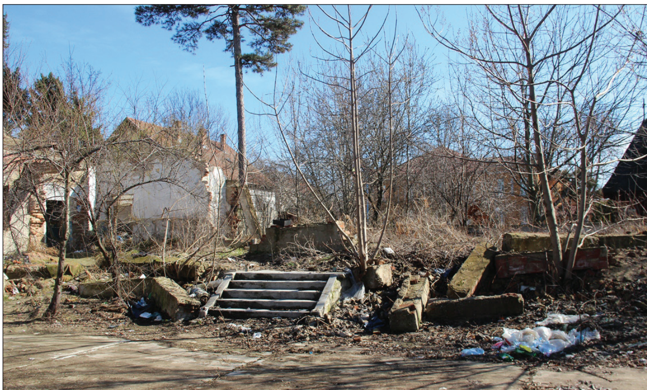
Figure 18: Former military buildings, currently in decay (Source: the authors).
