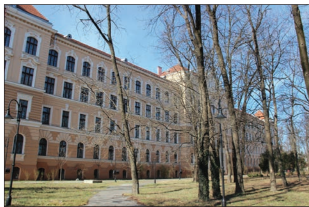
Figure 7: The front of the former the Royal Cadet School, the current location of the Bihor County Museum (Source: the authors).
