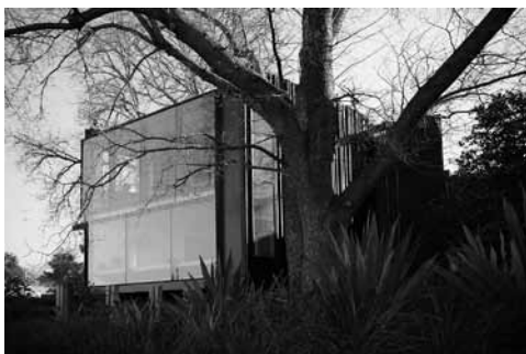
Hiša Kew, dolina Yarra Valley, Avstralija, dokončana 2000. Kew House, Yarra Valley, Australia, completed in 2000.
