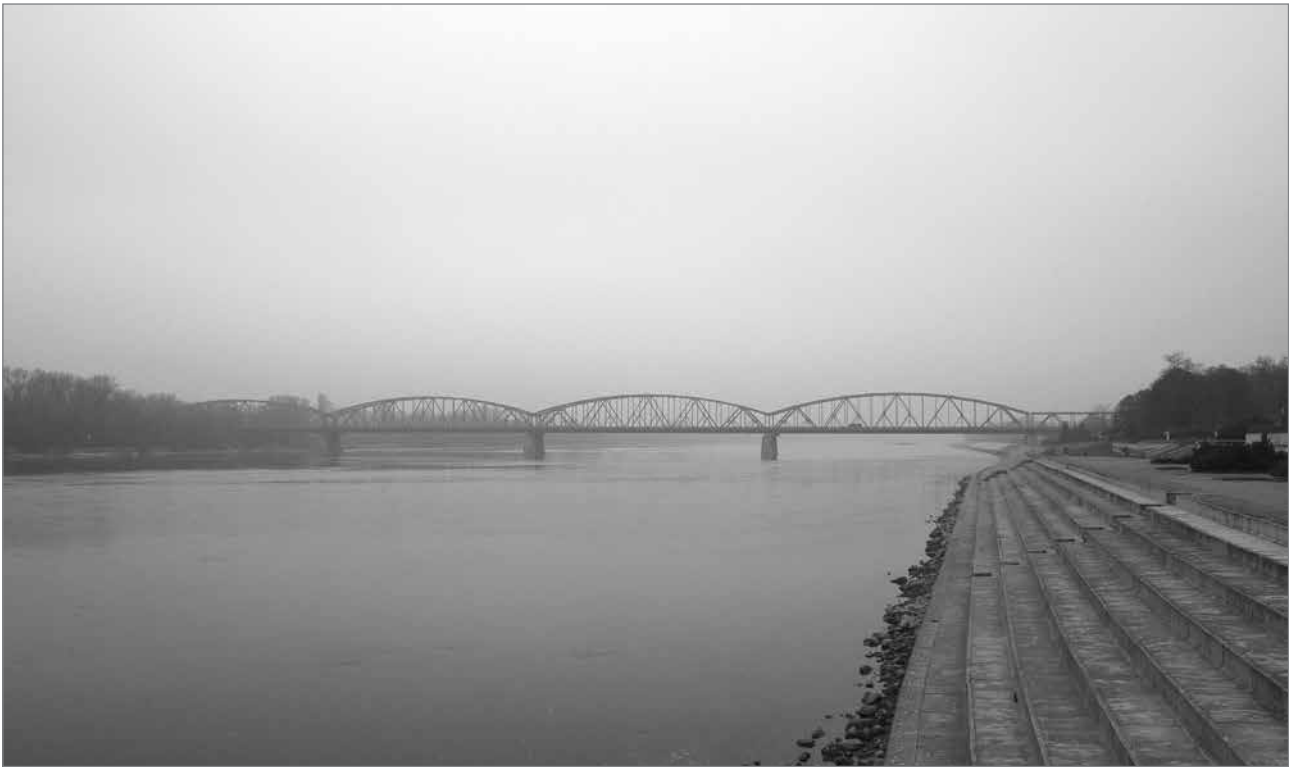
Figure 6: Main city bridge (photo: Rodrigo Rudge Ramos Ribeiro).
