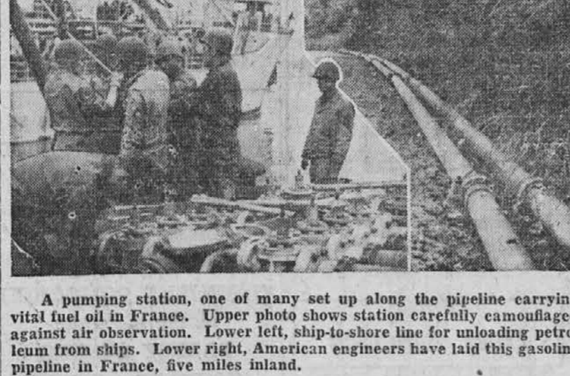
A pumping station, one of many set up along the pipeline carrying vital fuel oil in France. Upper photo shows station carefully camouflaged against air observation. Lower left, ship-to-shore line for unloading petroleum from ships. Lower right, American engineers have laid this gasoline pipeline in France, five miles inland.
